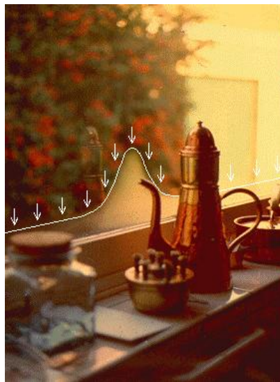
Figure 1. Surface condensation on single glazing.
