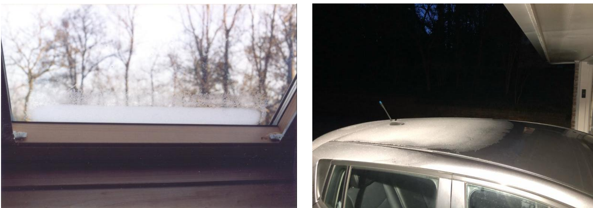
Figure 1. hoarfrost pattern on left) external side of a roof window and right) car partly parked in a carport
